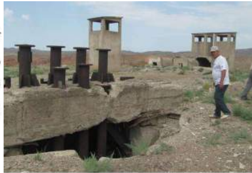
Tash-Komur free uranium mine entrance
